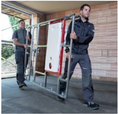
The finished installation wall is brought to the construction site; with the necessary mounting materials, of course.
