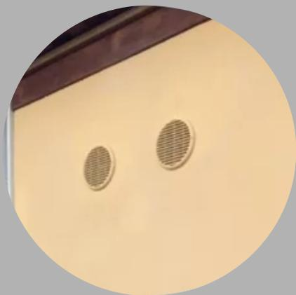
The flexible grill is useful when you need to install the outdoor grill from inside ambient , for example at the second , third floor .
