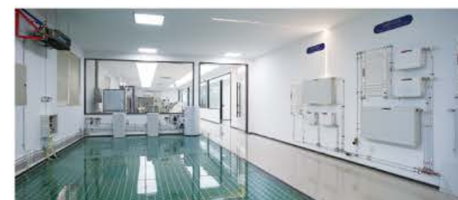
● System Connection Area
