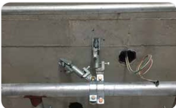
● Horizontal 4-way Sway Bracing
