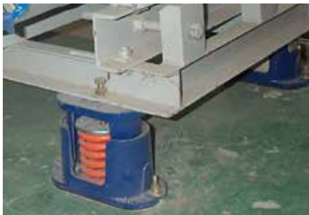
VENTILATION UNIT DETAIL
