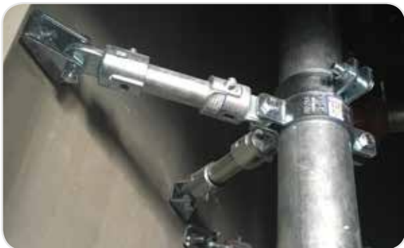
● 4-way Riser Sway Bracing
