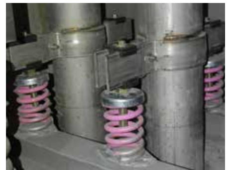
SPRING MOUNT INSTALL DETAIL
