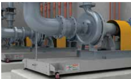
MULTI STAGE PUMP DETAIL
