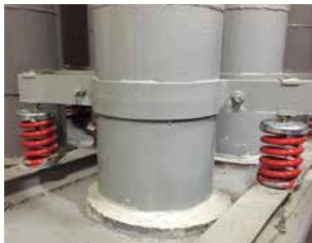
DOUBLE SUCTION PUMP DETAIL
