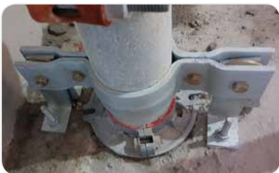
● 4-way Riser Sway Bracing (floor installation type)
