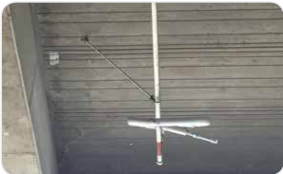
● Branch pipe Sway Bracing
