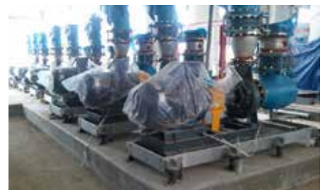
SINGLE STAGE PUMP DETAIL
