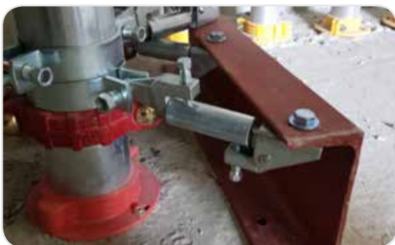
● 4-way Riser Sway Bracing (floor installation type)
