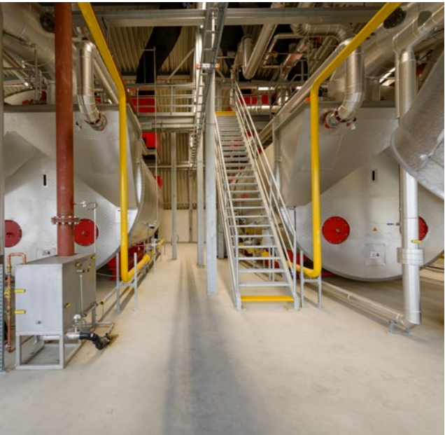
Flue gas heat exchanger ECO
