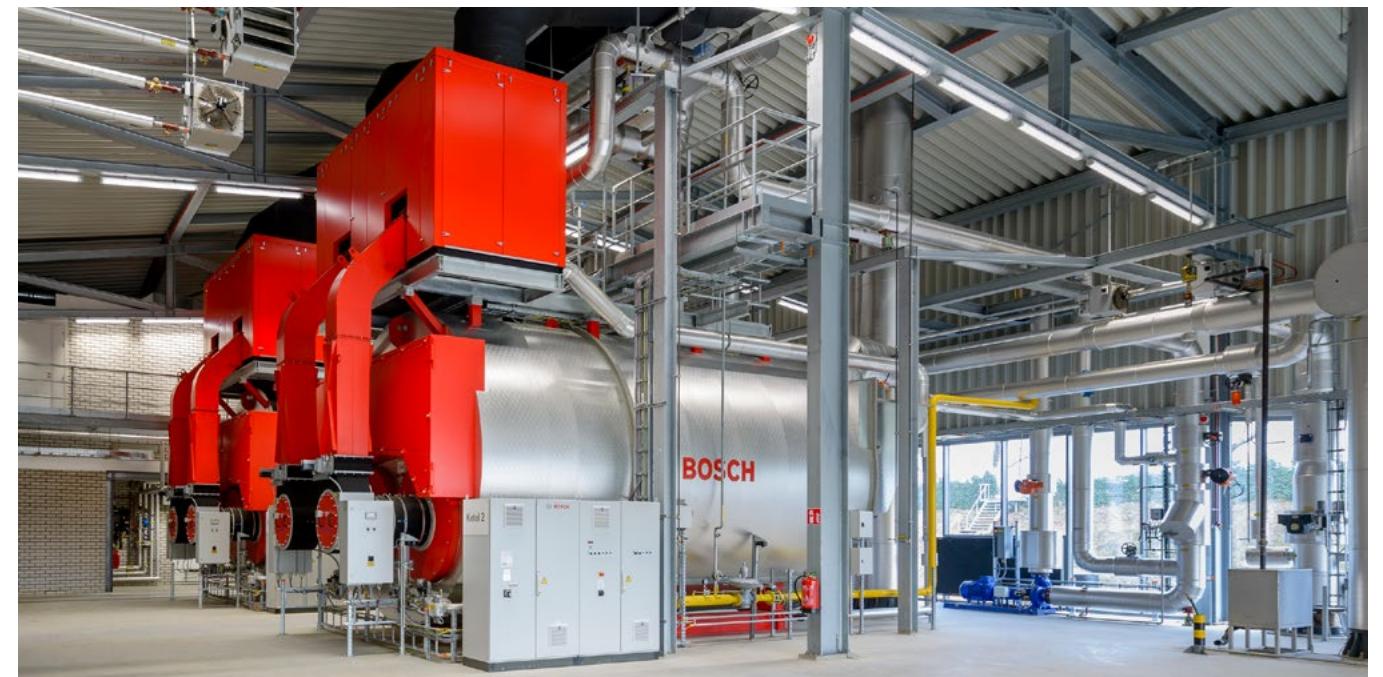
The NO x values are under 50 mg/Nm 3 at the customised boiler system in the Pieter Wiersma heating plant.
