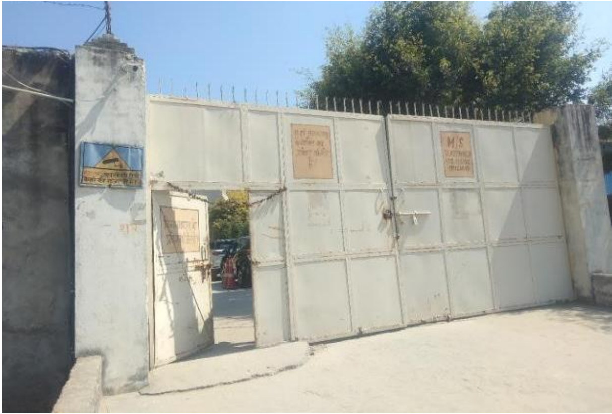
FACTORY MAIN GATE
