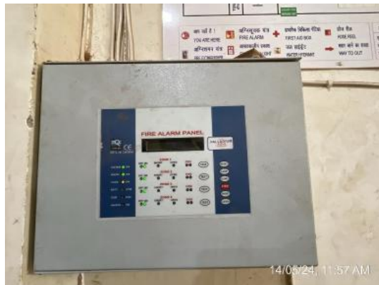
11.Fire Alarm Control Panel.jpg
