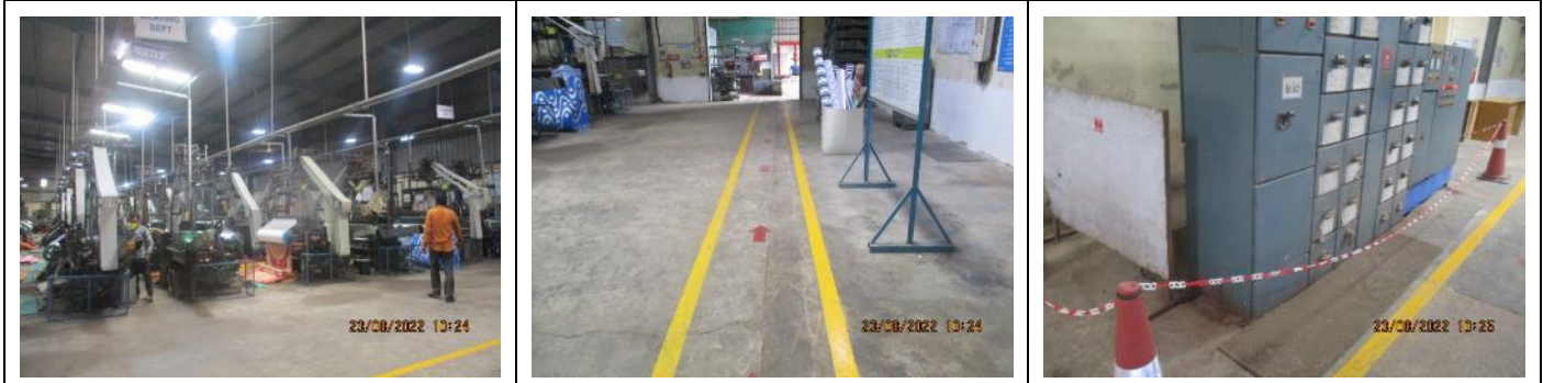
Loom shed Aisle marking done Rubber matt below electrical panel
