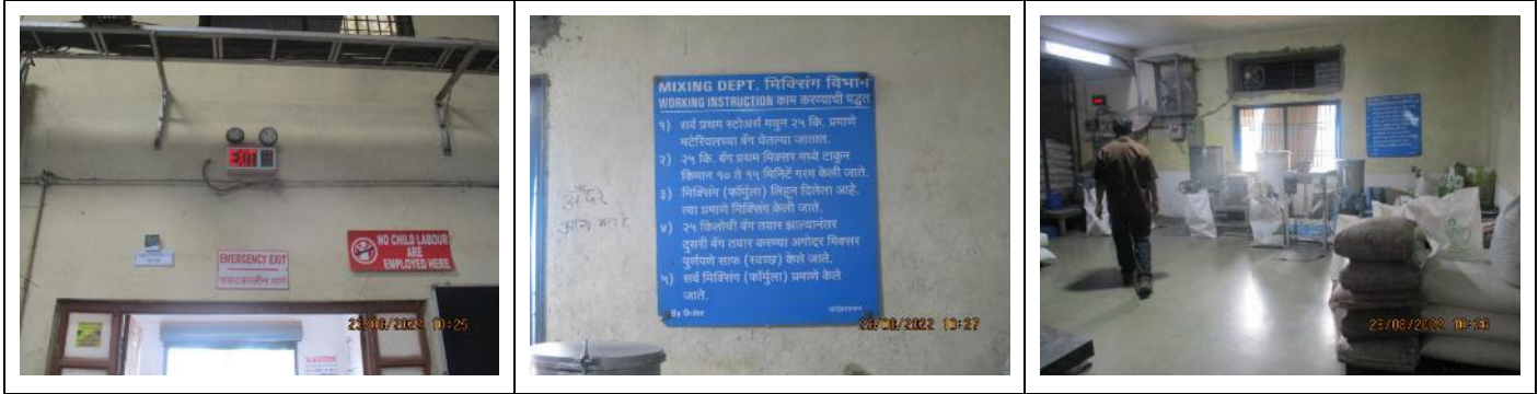
Emergency exit sign Safety instruction sign in mixing dept. Worker in factory setting
