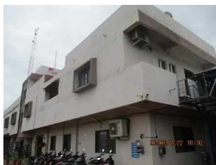
Facility building overview
